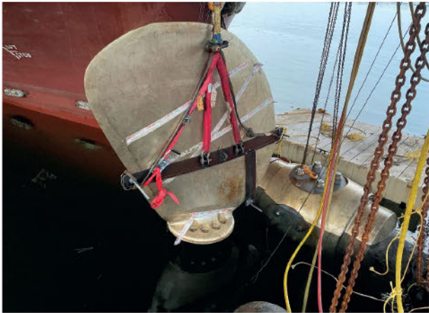
INSTALLING NEW PROPELLER BLADES, AFTER THE COFFERDAM HAS BEEN REMOVED
