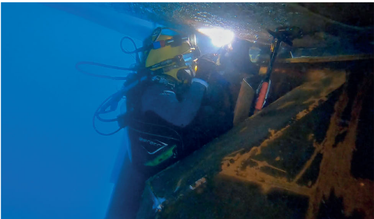
ONE OF HYDREX DIVERS WELDING A 45TON COFFERDAM IN PLACE
