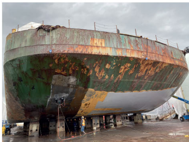
SHIPOWNERS ARE INCREASINGLY GOING TO ASK FOR EVIDENCE OF SHIPYARDS' ESG COMPLIANCE, FOR EXAMPLE THROUGH INVESTMENTS IN MORE ENVIRONMENT FRIENDLY ULTRA-HIGH PRESSURE (UHP) HYDRO-BLASTING SYSTEMS. SOURCE: EVERETT SHIP REPAIR
