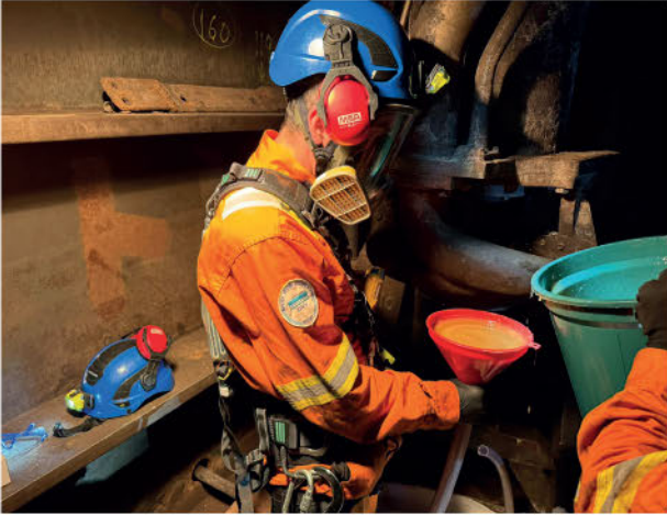
METALOCK ENGINEER CARRYING OUT AN FPSO REPAIR USING SPS TECHNOLOGY
