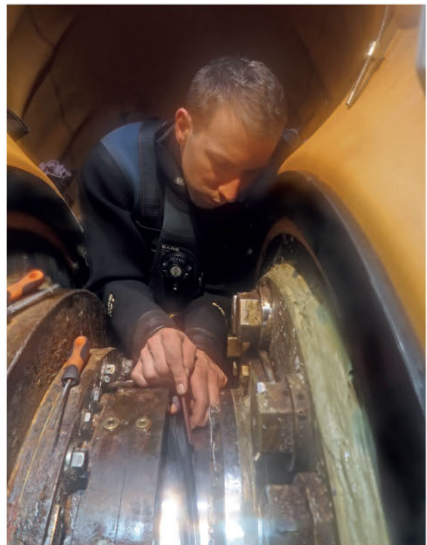
A DIVER-TECHNICIAN WORKING INSIDE A FLEXIBLE MOBDOCK
