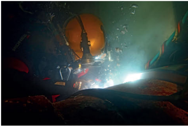
WELDING WORK ON A ROPE GUARD DURING A PROJECT IN TRINIDAD AND TOBAGO
